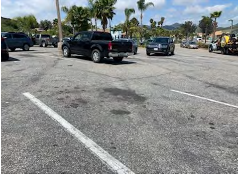
7. View north from central portion of property. Showing minor oil staining in parking stalls
