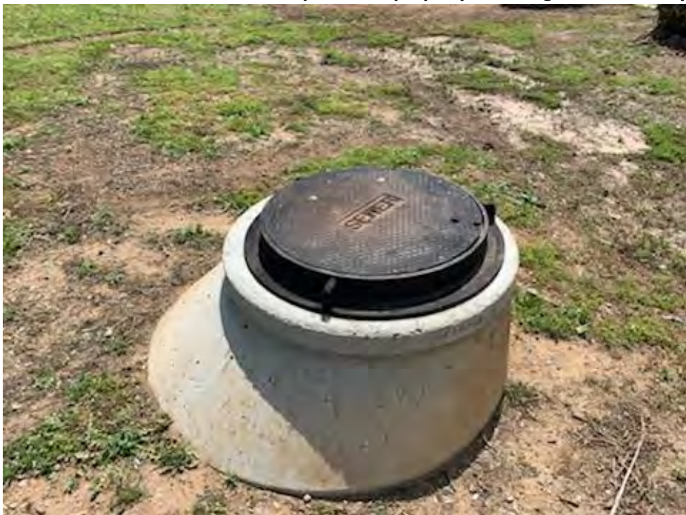
18. Near the northeast portion of the property. Showing sewer manhole.
