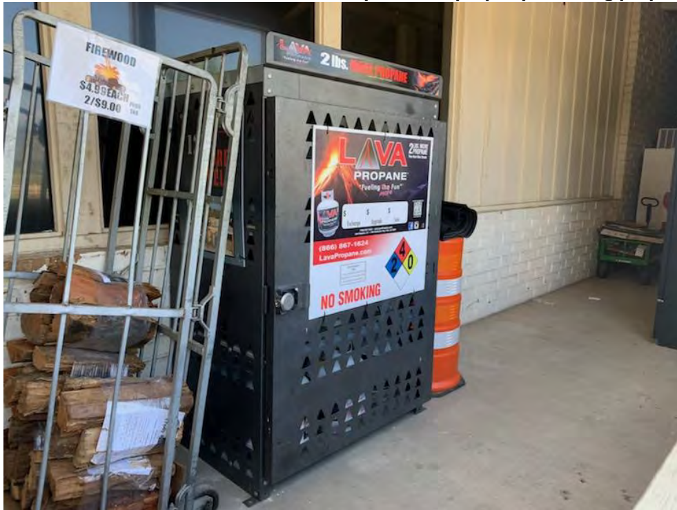
10. Central portion of property. Showing locked cage of propane gas tanks.
