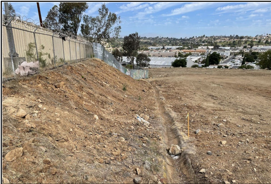
PHOTOGRAPH 2 Brow Ditch Along Southern Boundary, Looking West-Northwest
