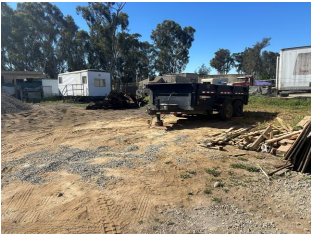
22. View of materials at the northern gravel lot.
