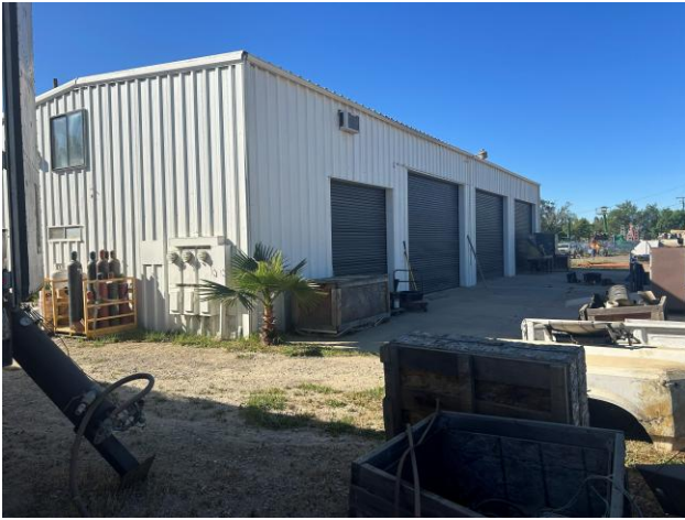
7. View of the former auto repair area at the northwestern portion of the Site.
