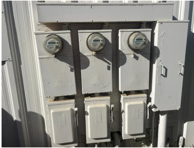
14. View of utility indicators.
