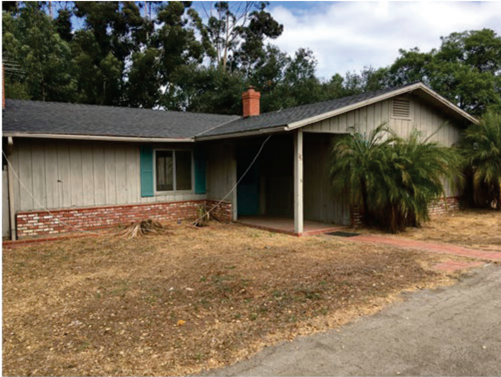
Figure 4: Overview of building. View North East.
