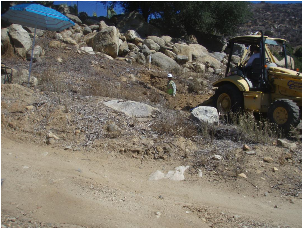
Test Pit TP-5 was excavated at the toe of the embankment fill slope.
