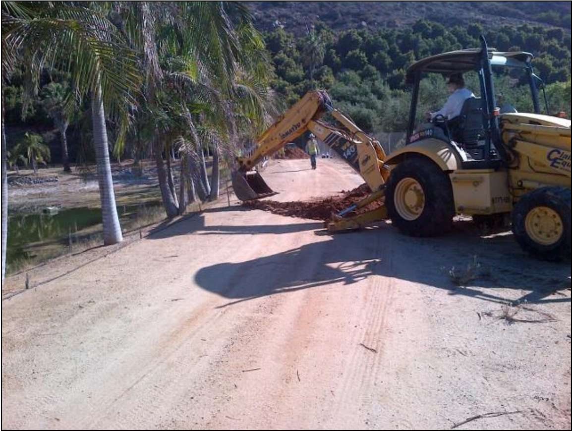
Backhoe test pits were excavated at the top of the embankment. This is Test Pit TP-2, looking east.
