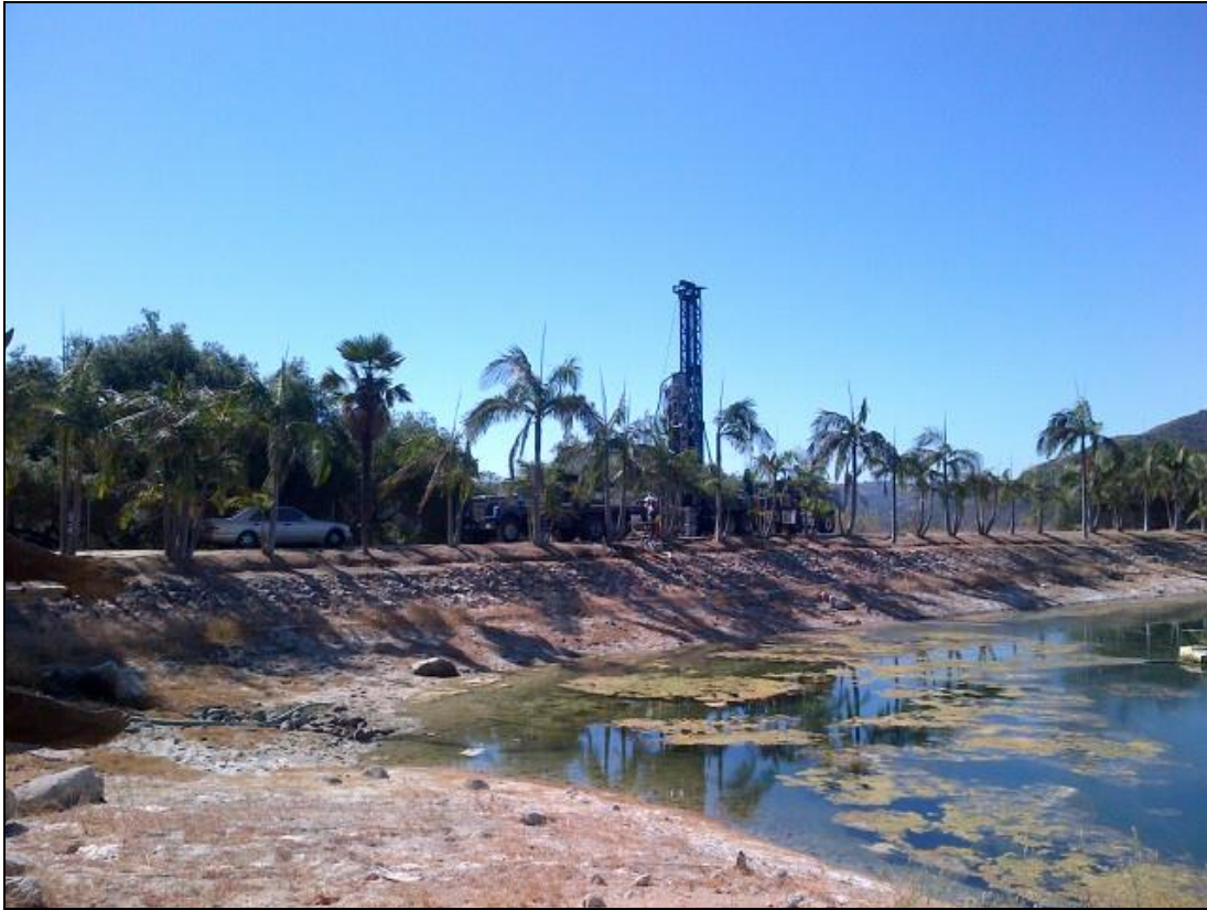
Becker hammer drill rig at Boring B-2. The reservoir level is about at the proposed final level.
