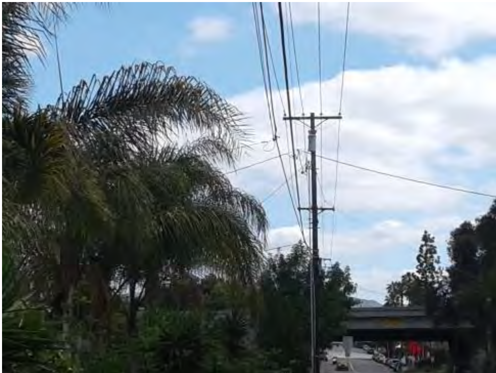
Photograph 18 – View of one of two (2) pole-mounted electrical transformers located in the vicinity of the subject property. None of the transformers observed showed any indication of potential leakage.
