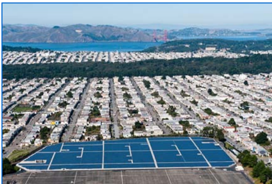
Recurrent Energy’s Sunset Reservoir solar array in San Francisco (photo courtesy Recurrent Energy)
