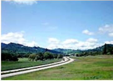
Route 101 - Mendocino County
