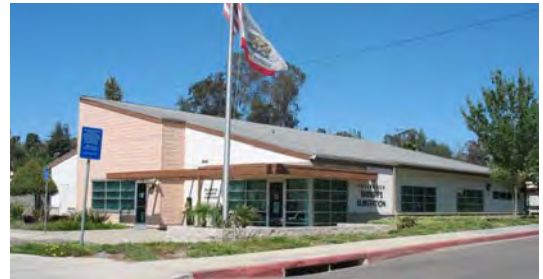
Fallbrook Sheriff substation
