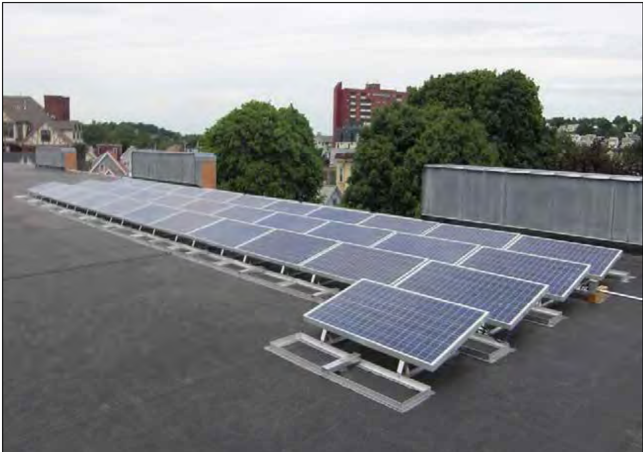
Figure 6: Example of a Roof-Mounted Solar PV System
