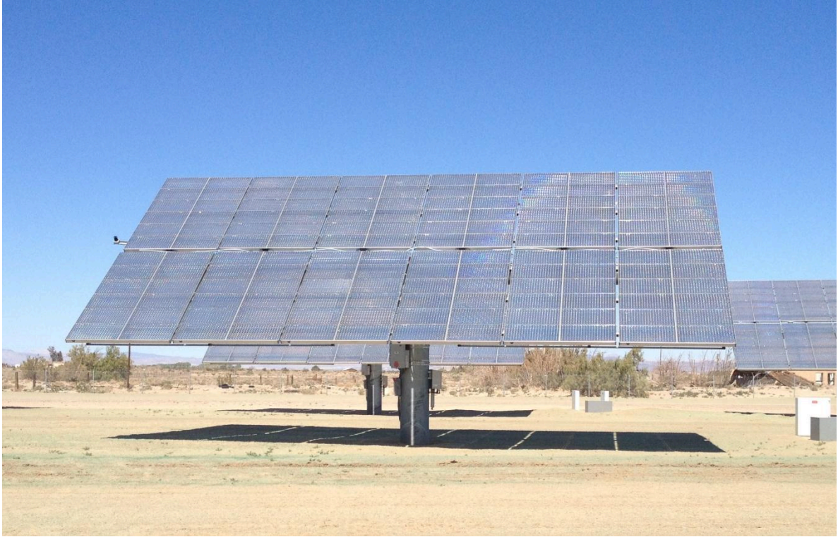
Figure 7: CPV Tracker
