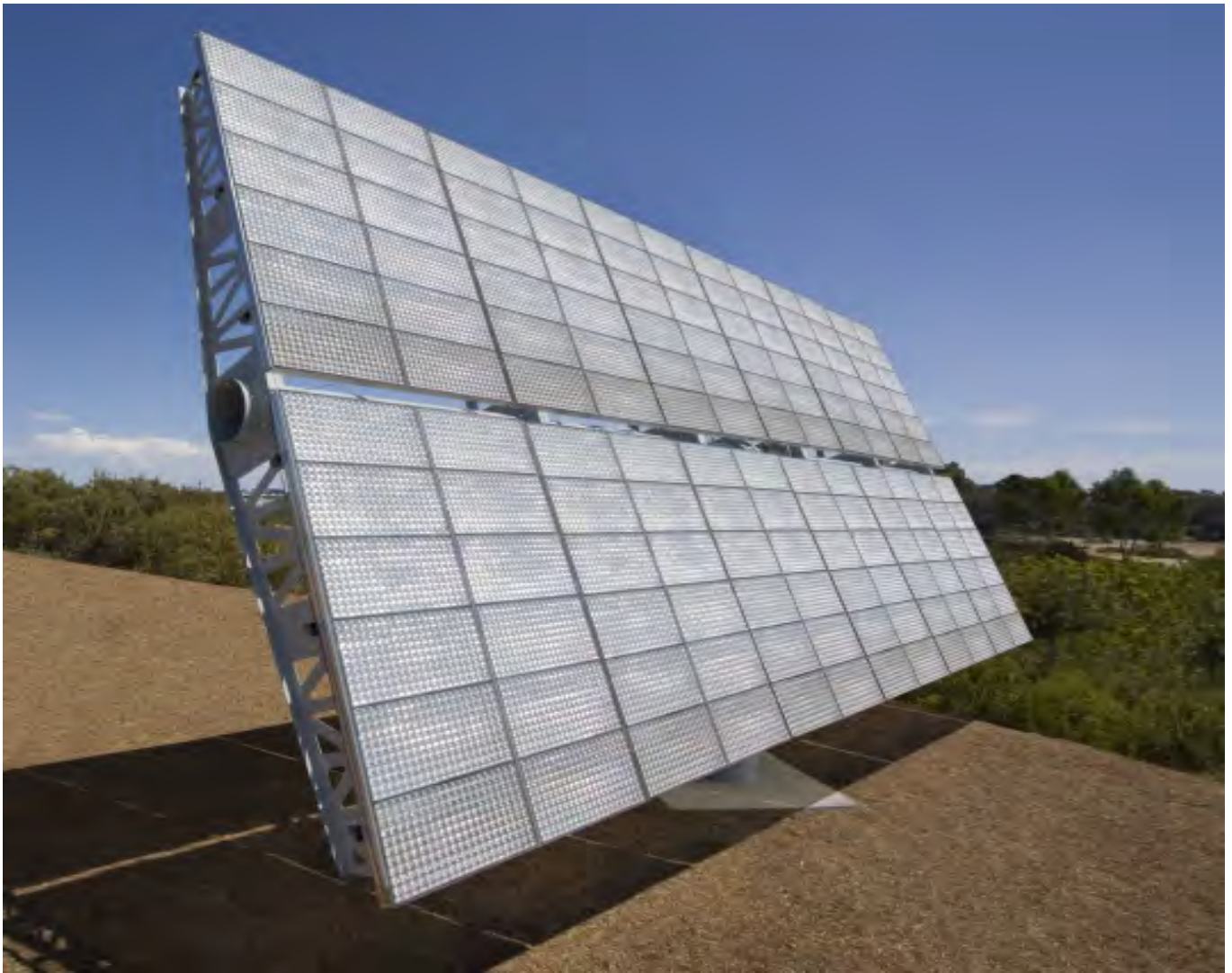
Concentrated photovoltaic (CPV) dual-axis tracking system
