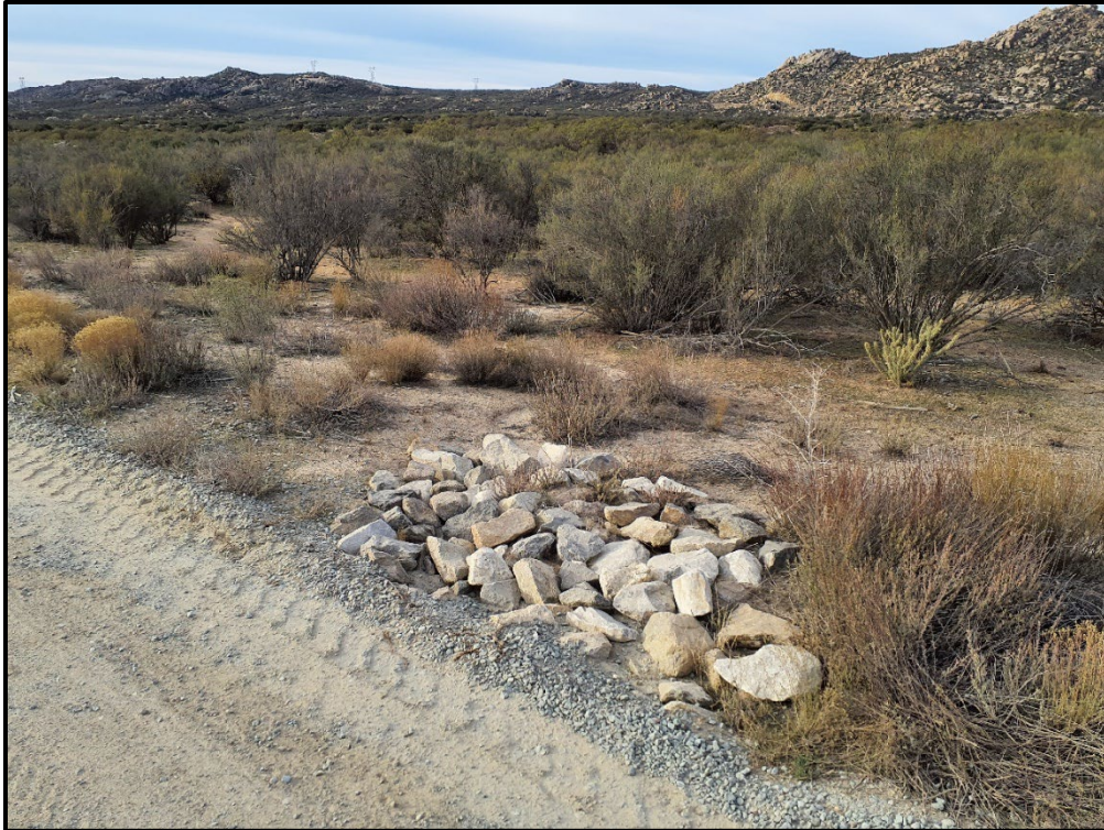
Photograph B43. Start of feature S60 from flow conveyed by road. Riprap is in place to reduce scour at side of the road. View facing downstream/southwest.
