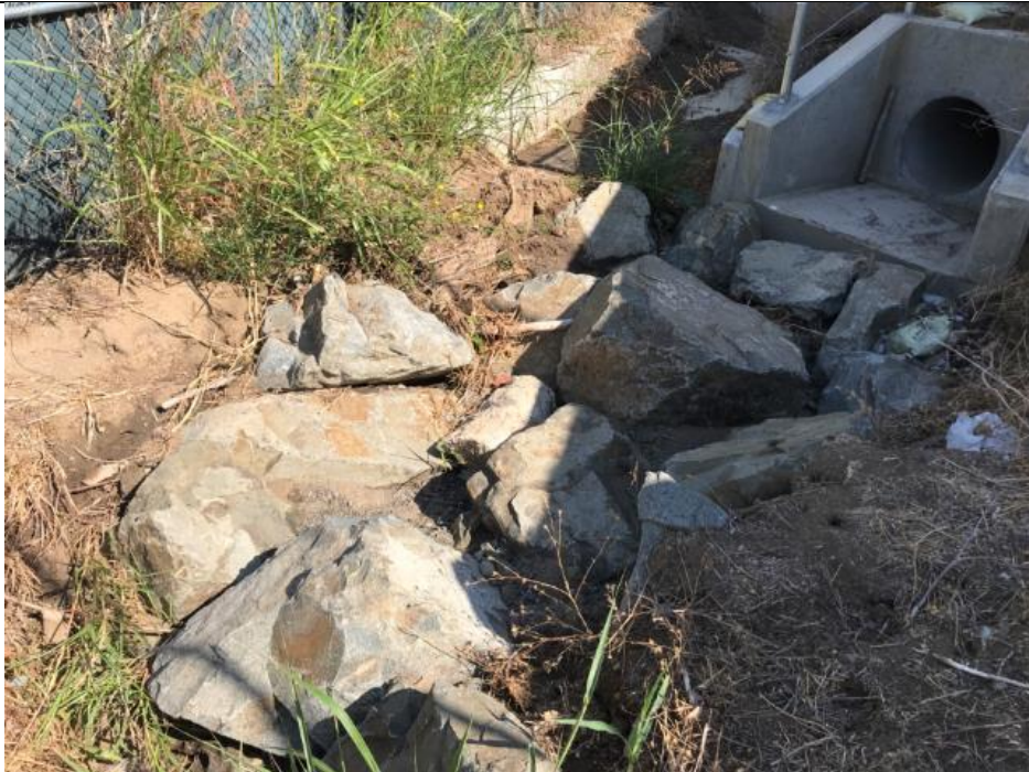
Photograph 2: (33.179, -117.216) North-facing view of the 4-foot-wide earthen-bottom channel on the eastern edge of the project site. This photo shows where sampling point NW-2 was taken to determine the presence of OHWM indicators. This photo also shows the approximately 3-foot-diameter concrete culvert that runs east under the train transportation corridor east of the project site and the concrete and rock riprap in the center of the earthen-bottom channel.
