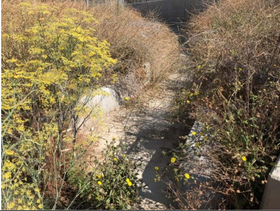
Photograph 5: (33.179, -117.216) North-facing view of the 5-foot-wide concrete-lined portion of the channel on the northeastern edge of the project site. This photo shows where sampling point NW-5 was taken to determine the presence of OHWM indicators.
