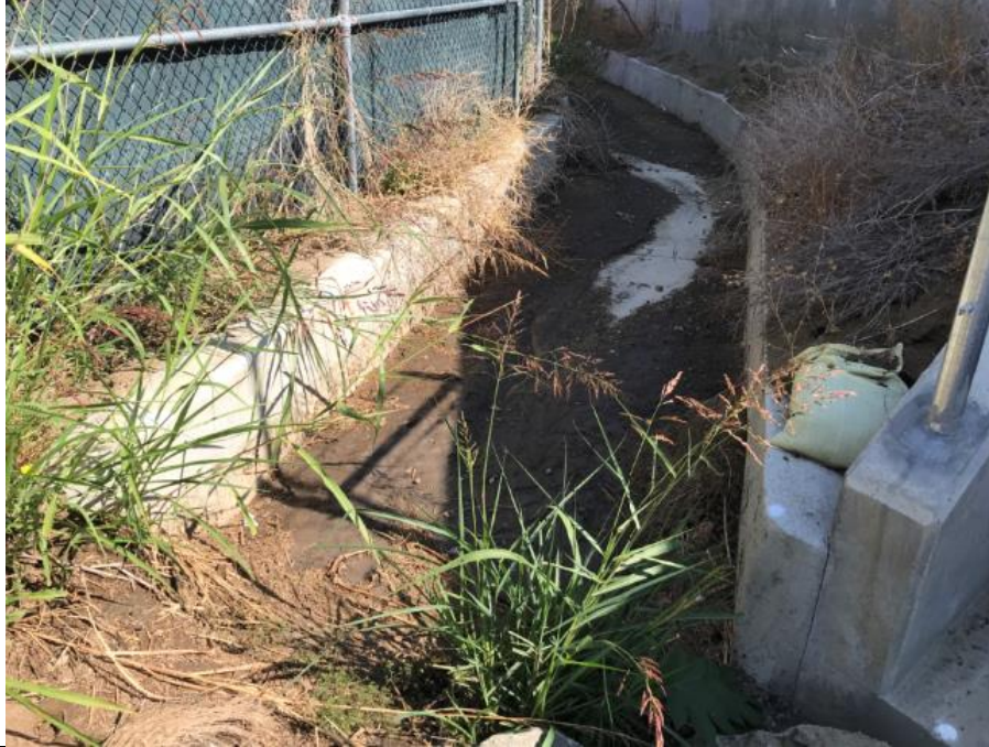
Photograph 3: (33.179, -117.216) North-facing view of the 4-foot-wide concrete-lined portion of the channel on the eastern edge of the project site. This photo shows where sampling point NW-3 was taken to determine the presence of OHWM indicators. The approximately 3-foot-diameter concrete culvert that runs east under the train transportation corridor east of the project site is shown on the right side of the photo.
