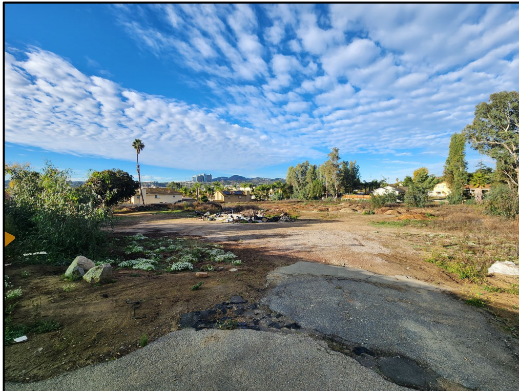
Plate 1: Overview of the project, facing west.
