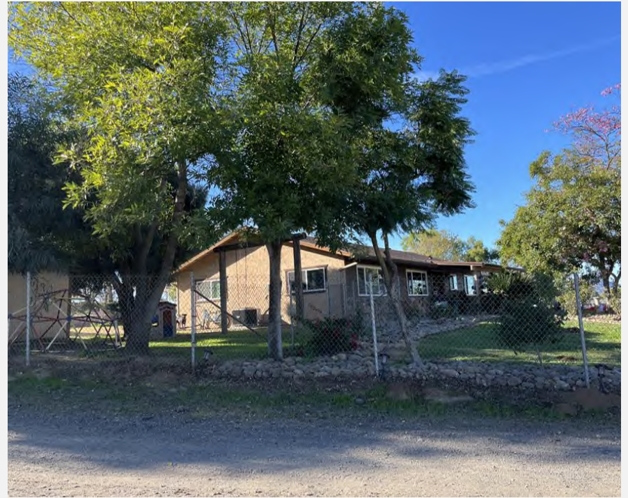
Photo 6. Photo location 1, looking southwest
