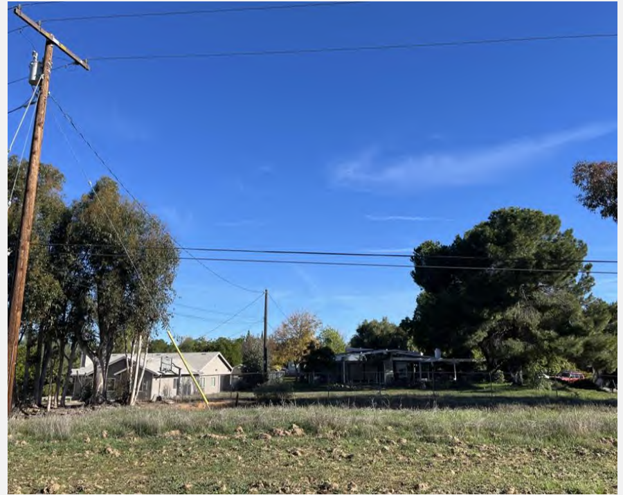
Photo 18. Photo location 3, looking northeast
