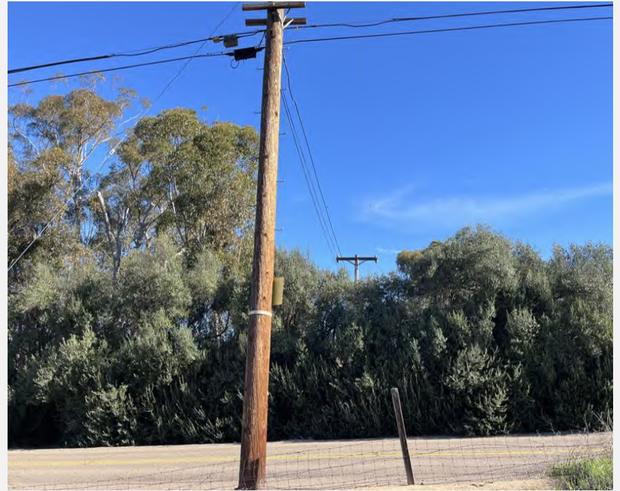
Photo 26. Photo location 4, looking northeast
