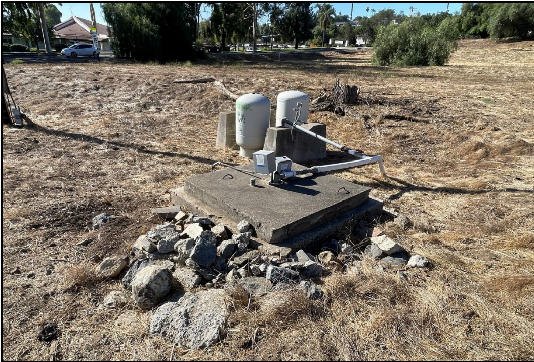
PHOTOGRAPH 7 Overview of Updated Well Structure, Looking South
