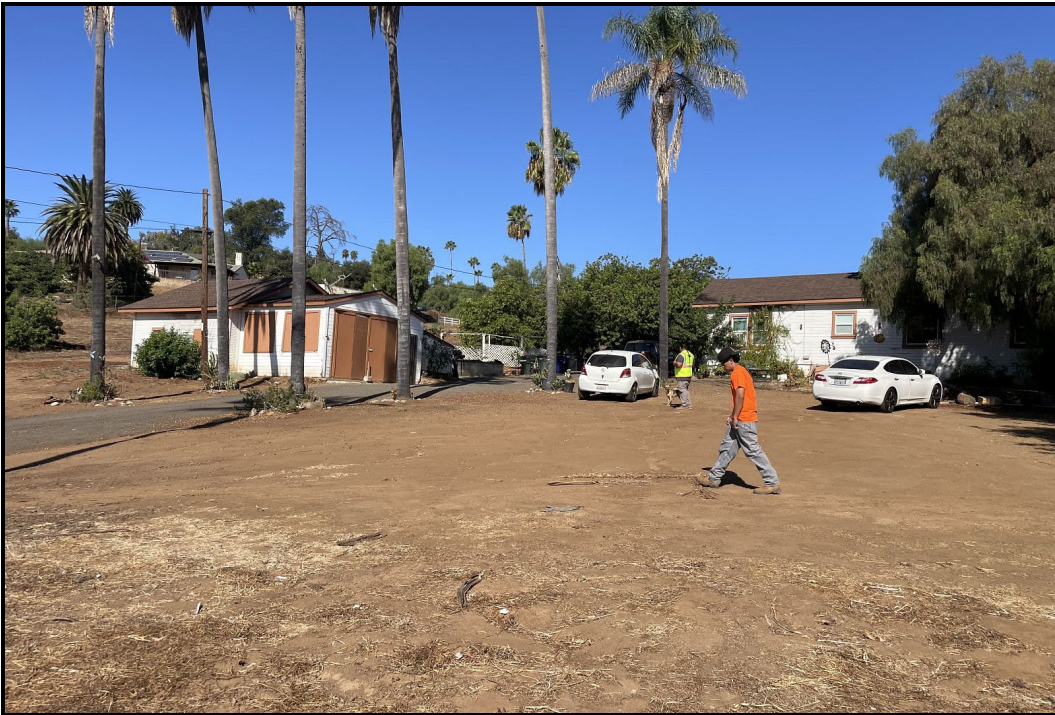
PHOTOGRAPH 5 Overview of Single-Family Residence and Garage, Looking Northwest
