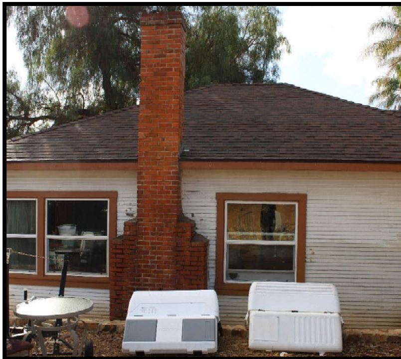
Figure C-5 Exterior of 830 Idaho Street Showing Chimney. Looking South
