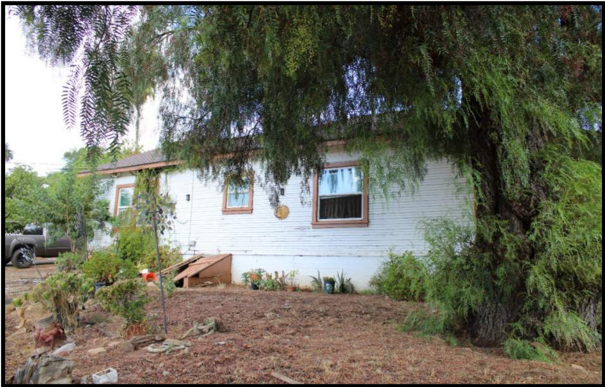
Figure C3 Exterior of 830 Idaho Avenue Looking Northeast
