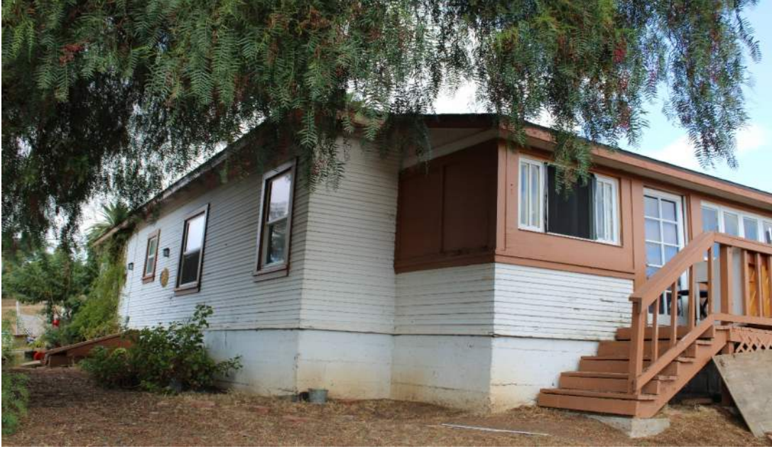
Figure C2 Exterior View Looking Northeast
