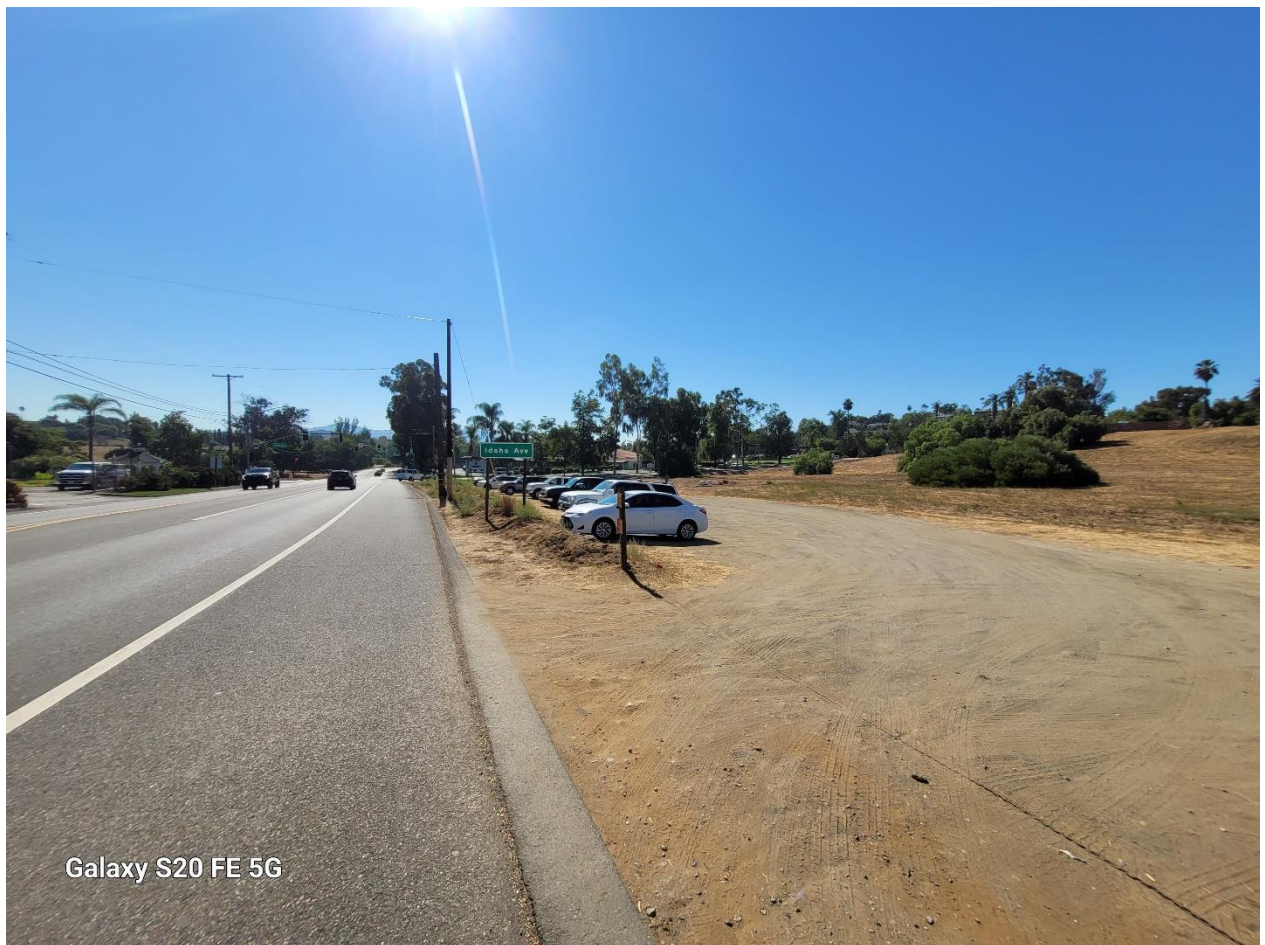
Photograph 40: View of San Pasqual Valley Road and onsite parking area looking southeast.
