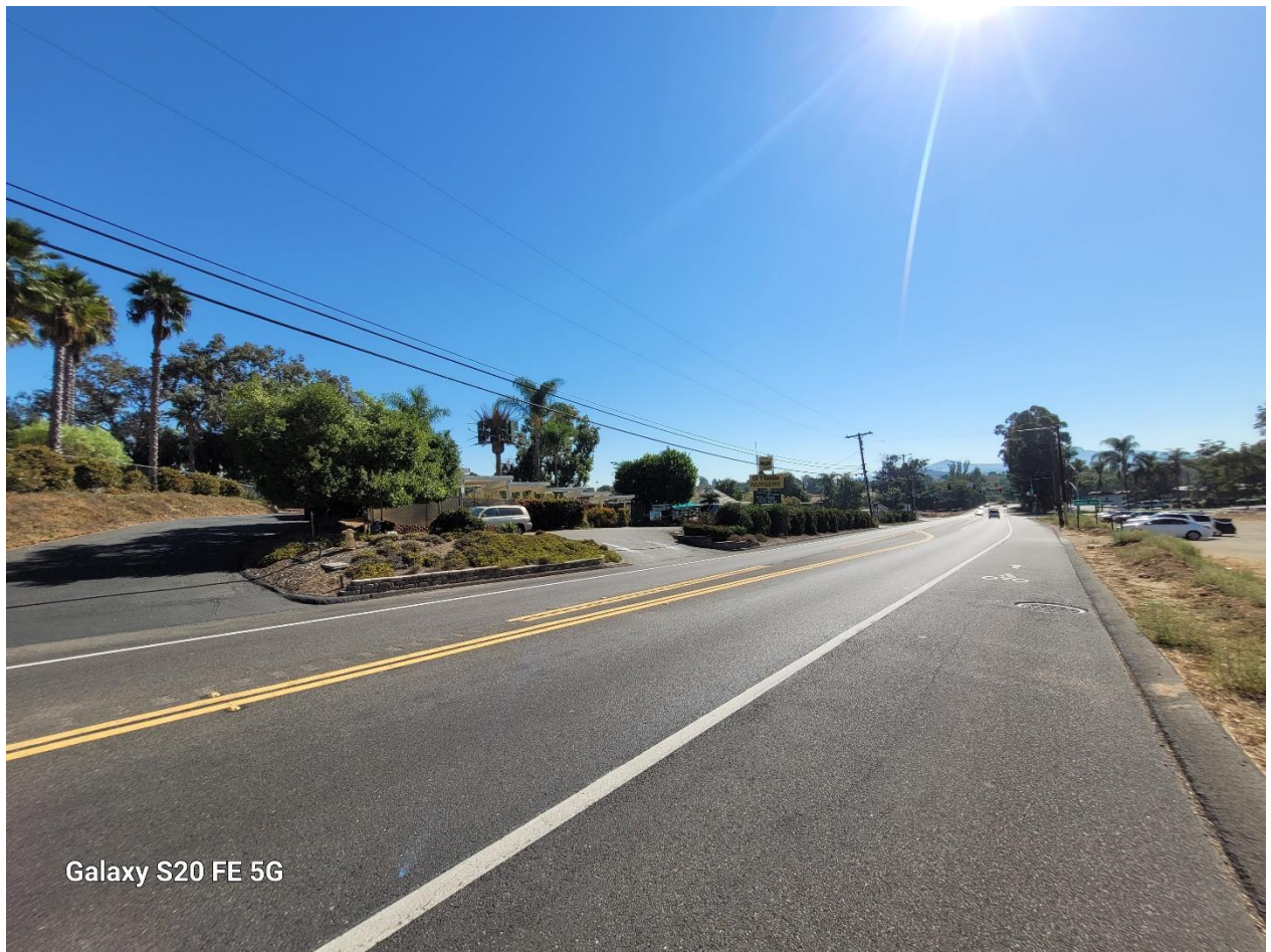
Photograph 39: View of San Pasqual Valley Road from corner of site at access road looking southeast. Note round storm drain inlet in road on right side of view.
