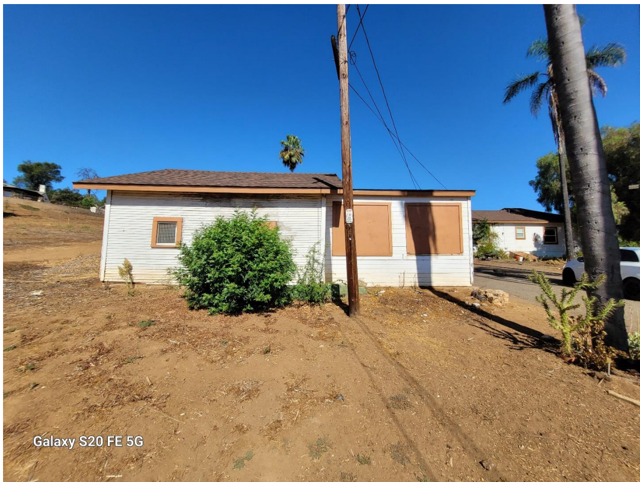
Photograph 5: View of south side of garage looking north.
