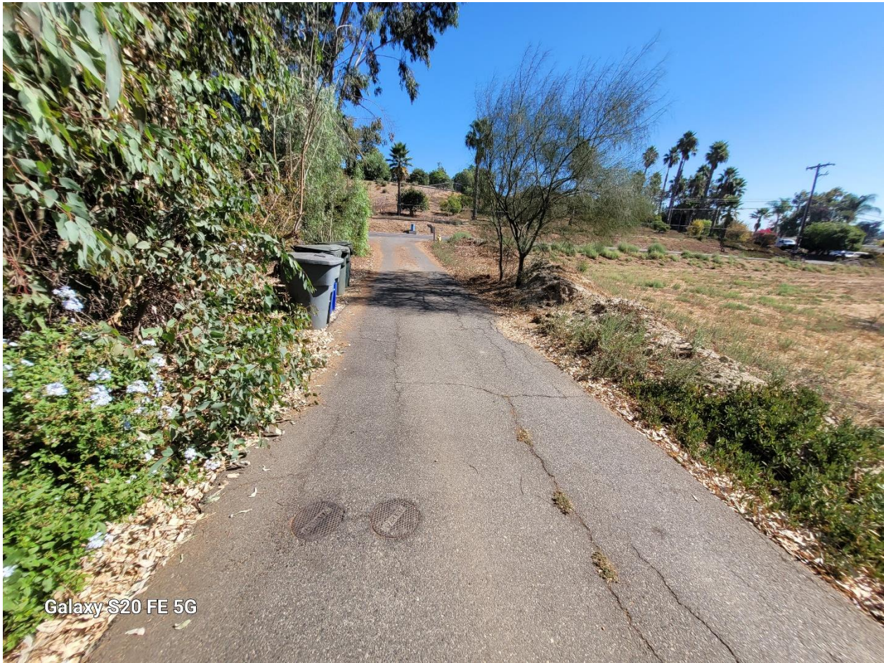
Photograph 35: View of access road along northeast area of site looking northeast toward San Pasqual Valley Road.
