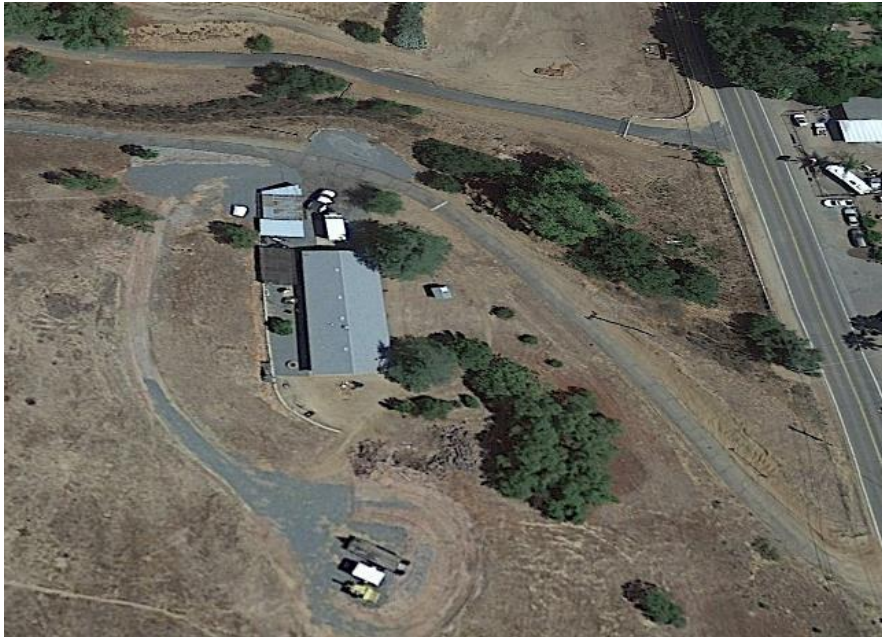
1985 Aerial Image of the Remainder Lot and its Defensible Space Provisions
