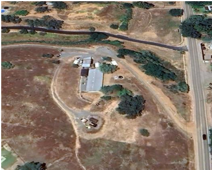
2023 Aerial Image of the Remainder Lot and its Current Defensible Space Provisions
