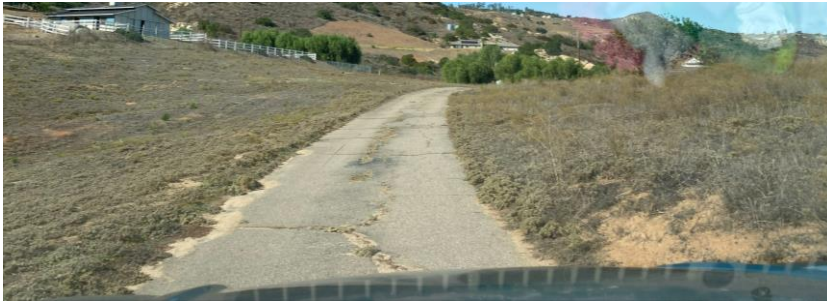
Typical Driving Surface of Existing Driveway, Looking North from Proposed Parcel 3
