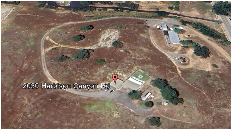
Existing Project Site Roadway System
