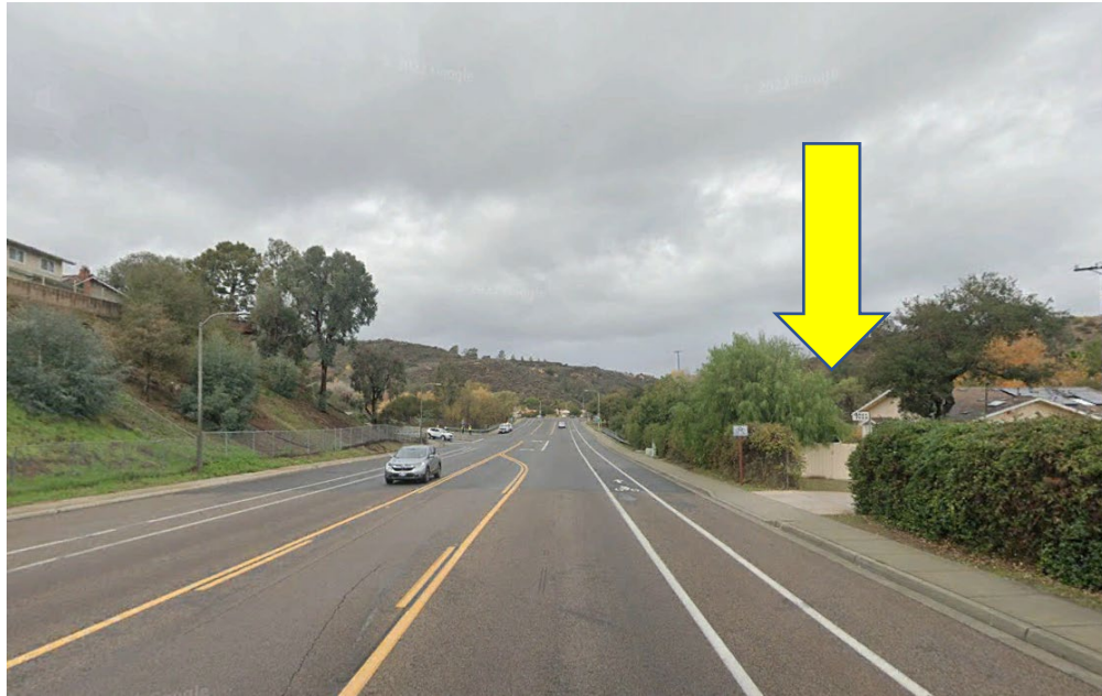
Northern Evacuation Route on Los Coches Road (YELLOW arrow – Project Site)
