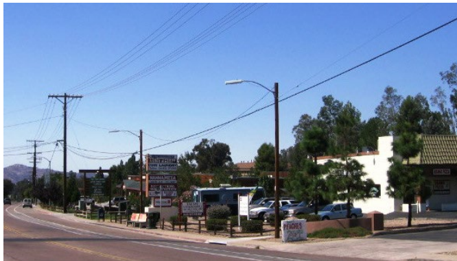
Alpine Boulevard serves as the primary circulation route in the village of Alpine
