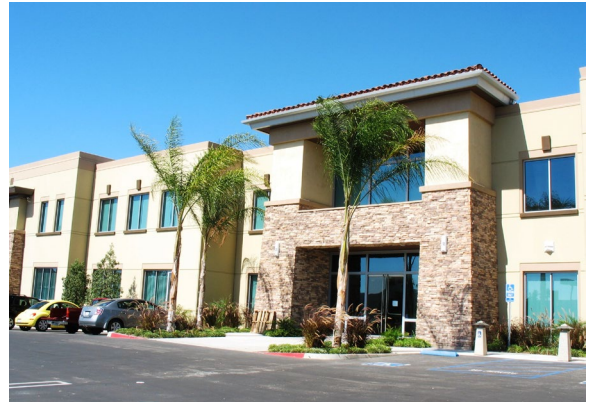
Office complex in Rancho San Diego
