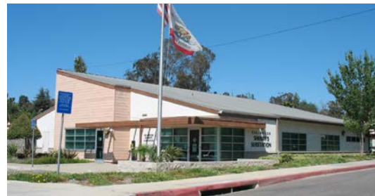
Fallbrook Sheriff substation
