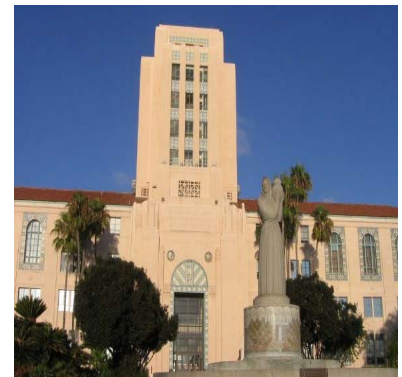
County Administration Center
