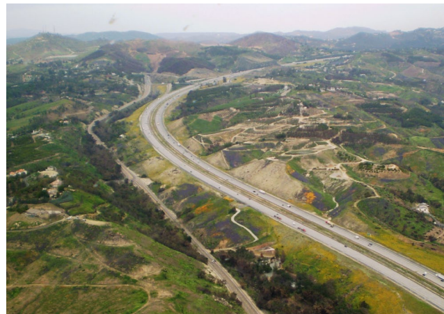
Interstate 15 looking north
