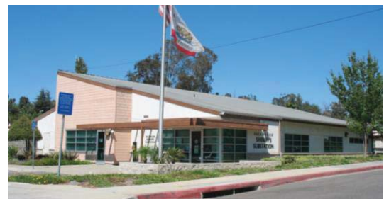
Fallbrook Sheriff substation
