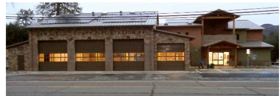
Fire Station in Pine Valley
