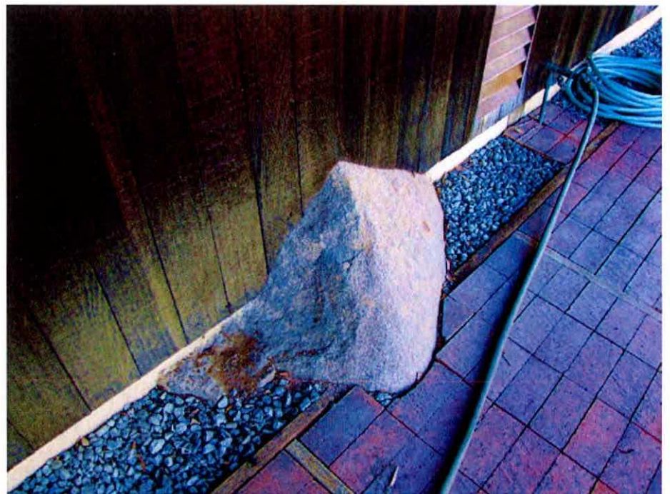
Photo 15: View of a boulder integrated into the foundation at the north facade basement level.
