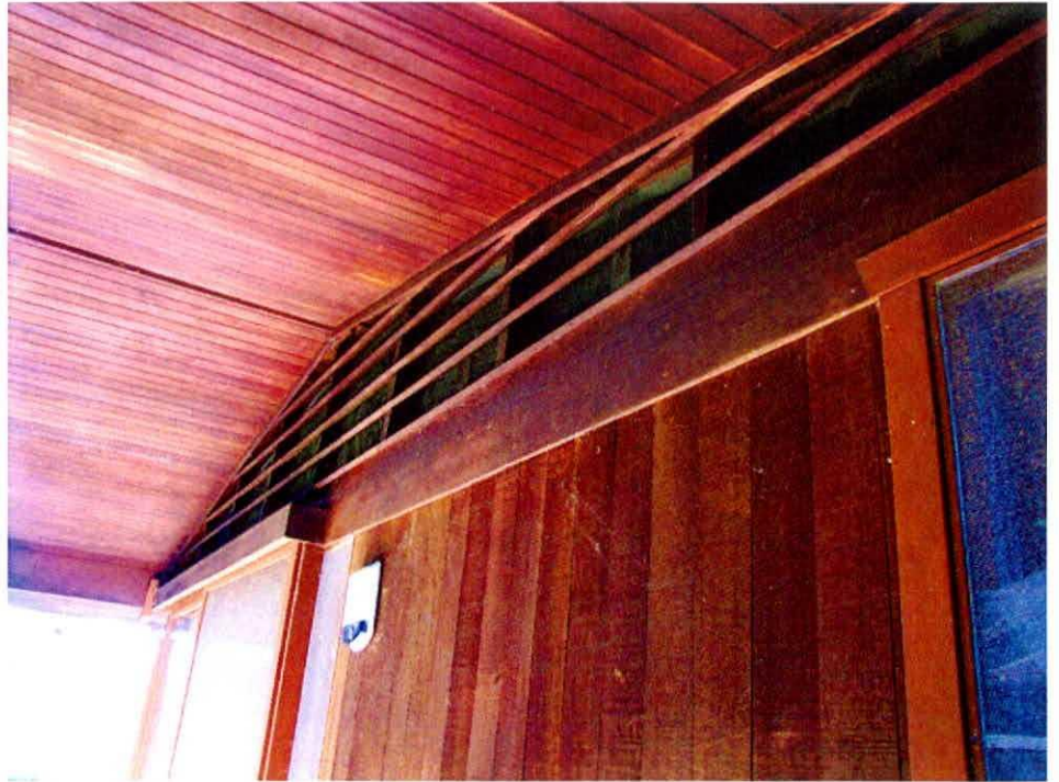
Photo 22: Typical view of the redwood soffit and 5' eave overhang around the perimeter of the house, and showing additional louvered gable vents.
