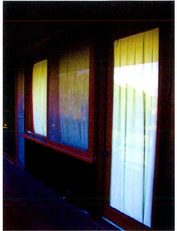
Photo 12: Typical fixed and sliding units and typical single entry door at the north facade.
