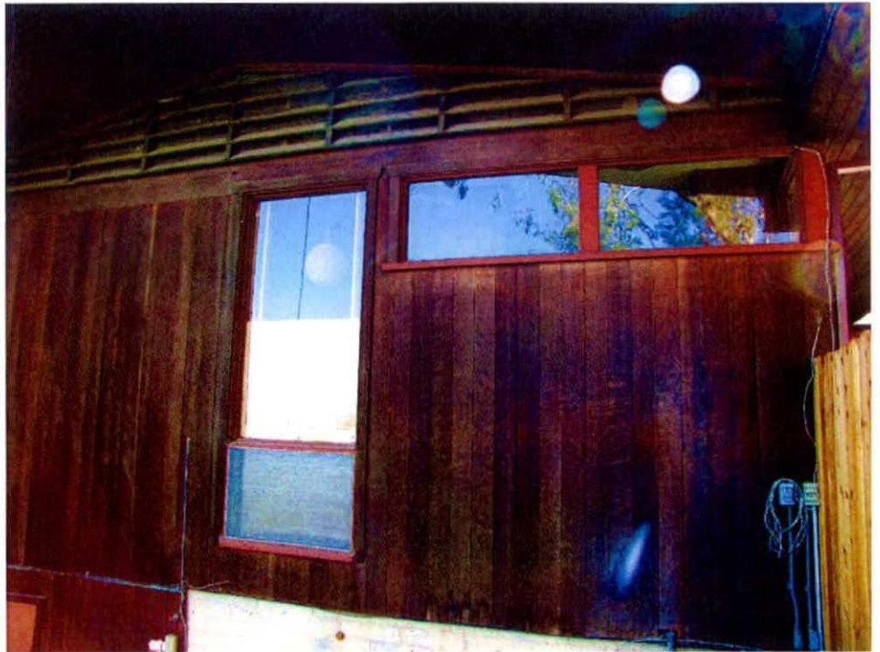
Photo 18: View of the west facade main level including fixed units, louvered glass unit, and louvered gable vents with built-in insect screens.
