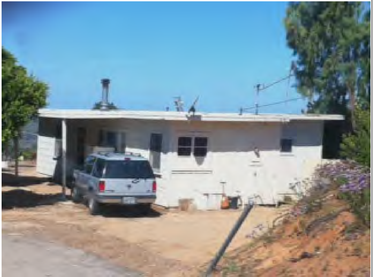
View of residence – looking WNW
