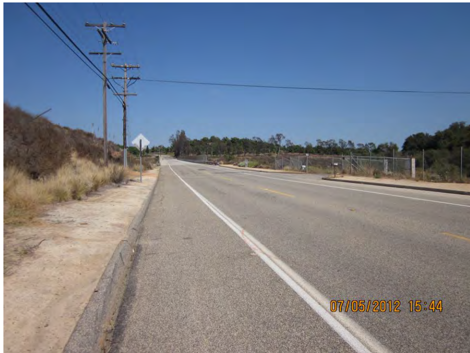
Photograph 2 – East view along the northern edge of West Lilac Road. Concrete pavement in background is the I-15 overpass. Note strip storm drain inlet inside of asphalt curb in left foreground.
