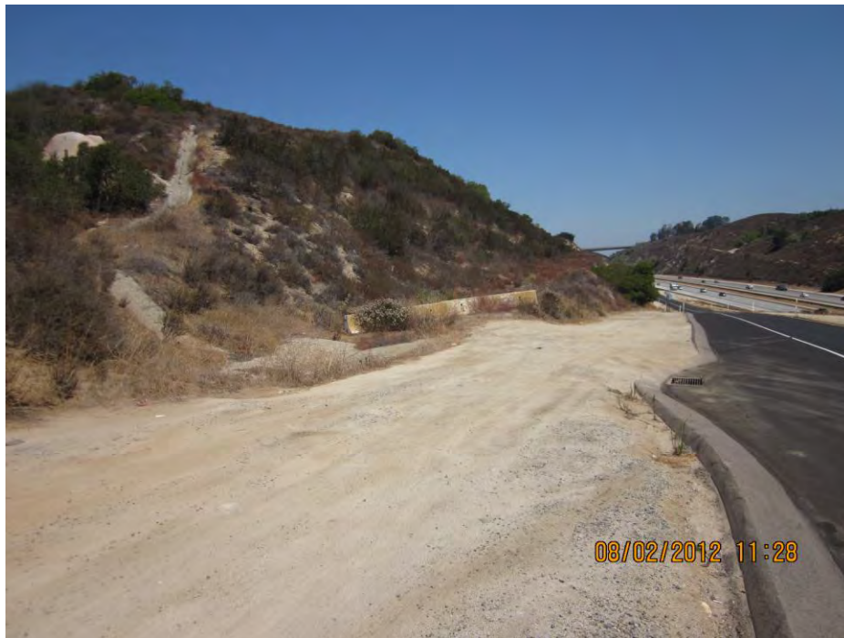
Photograph 4 – North view along the southbound I-15 off ramp for Old Highway 395. Note 3 drainage structures (i.e., grate inlet; concrete-pave inlet basin; and concrete-paved swale) near northerly end of proposed improvement area.
