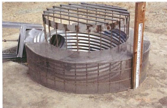
Figure 1 Example of Extended Detention Outlet Structure
