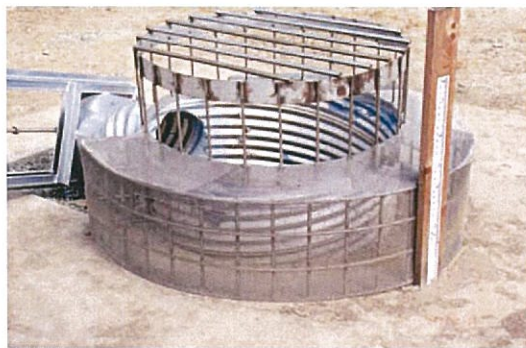
Figure 1 Example of Extended Detention Outlet Structure
