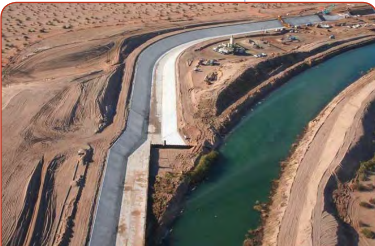
The AAC lining project makes 67,700 AF of Colorado River water per year available for allocation to the Water Authority and San Luis Rey Indian water rights settlement parties.
