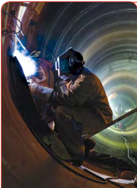
As part of the Asset Management program, workers weld the joints between pipe sections.
