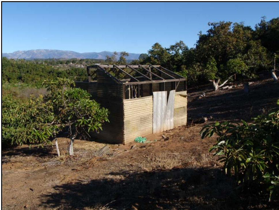
Photograph 8 – View of a second wooden shed in the southwest portion of the subject property. View is to the northeast.
