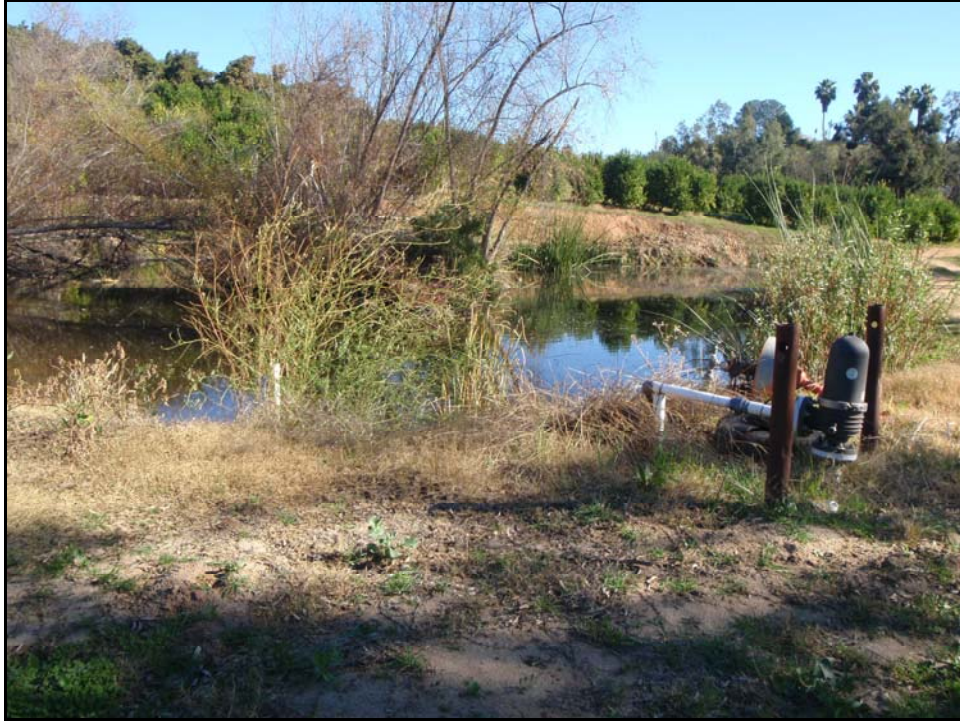
Photograph 3 – View of the small man-made pond located in the southern of the subject property. Note the pumping equipment on in the foreground.
