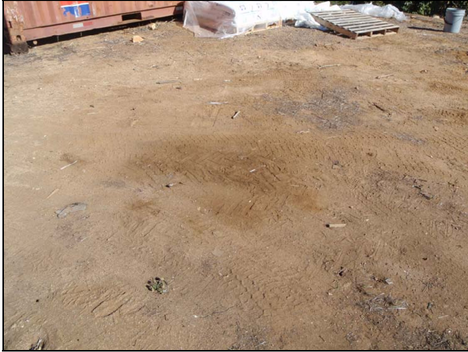
Photograph 5 – View of stained soil south of the metal storage container located on the southwest corner of site. Connex storage container and pallets of fertilizer also in view.
