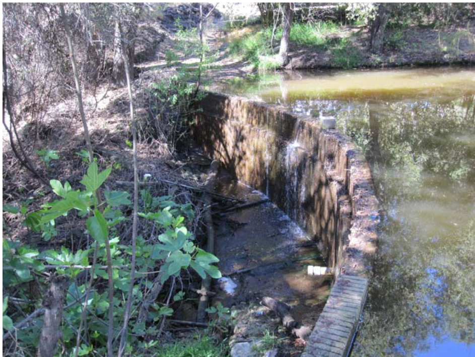
Photograph 6 – View of the dam located on the southern end of the pond.
