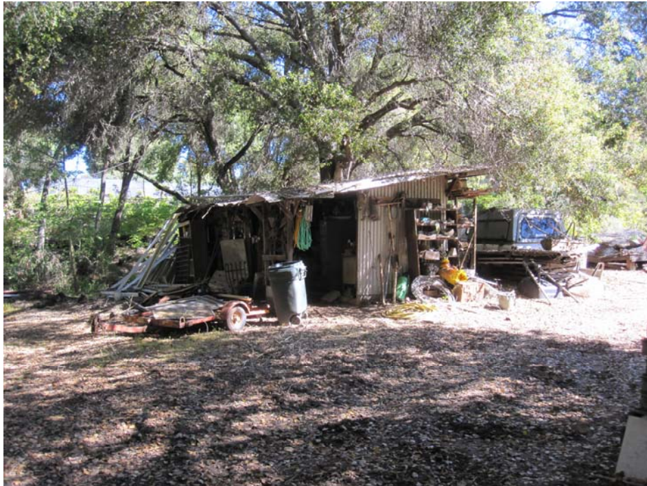
Photograph 7 – View of the maintenance shed located within the central portion of the site.
