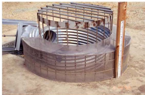
Figure 1 Example of Extended Detention Outlet Structure
