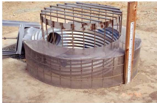
Figure 1 Example of Extended Detention Outlet Structure
