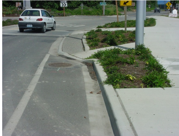
Picture 1: Angled Bike Ramp
