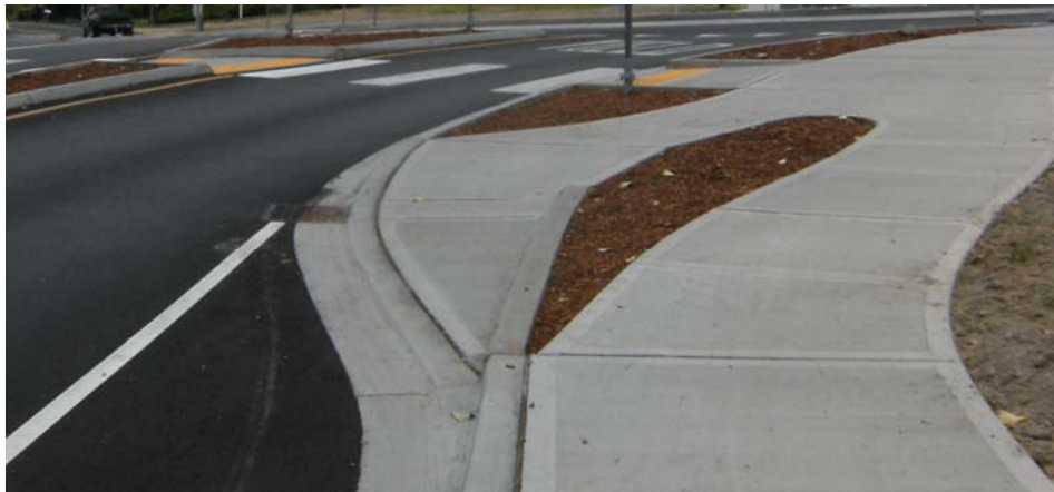
Picture 4: Angled Bike Ramp
