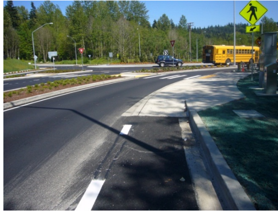
Picture 3: Ramp with Minimal Landscaping Buffer
