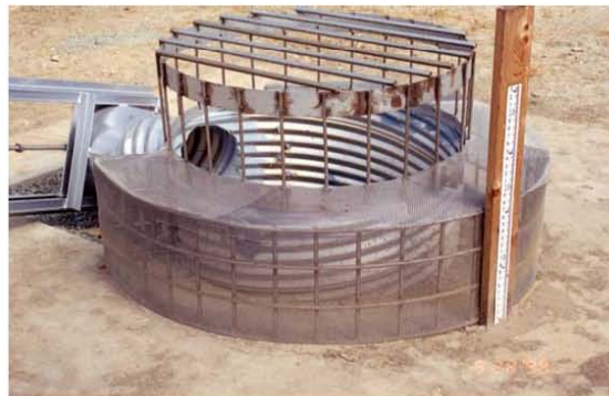
Figure 1 Example of Extended Detention Outlet Structure
