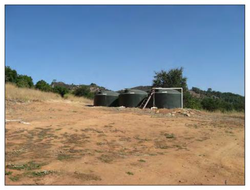
Photograph No.19 View to the northwest of the three 5,000-gallon polyethylene ASTs on site parcel 232-013-02.
