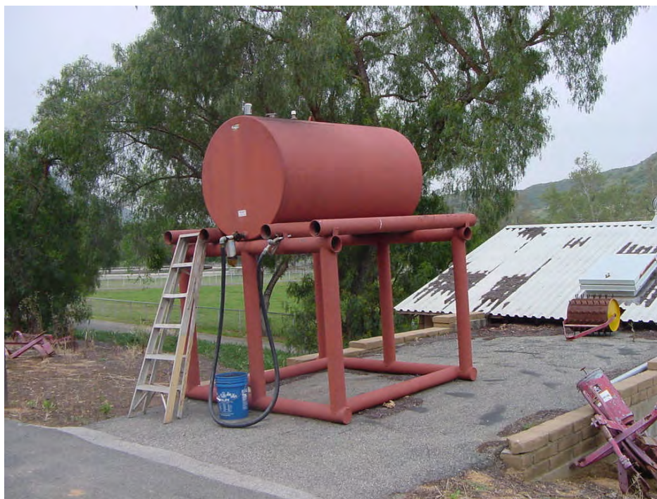
Photograph #2 Gasoline AST adjacent to hazardous materials storage garage.
