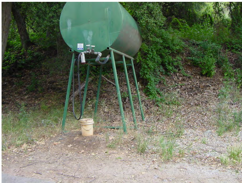
Photograph #3 Diesel AST with minor soil staining in west-central portion of the Site.
