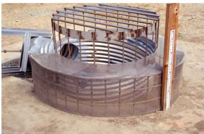
Figure 1 Example of Extended Detention Outlet Structure
