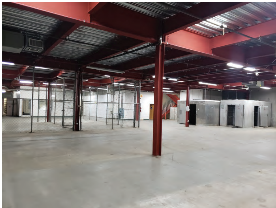
Photograph 6: View within the warehouse and cold storage rooms.
