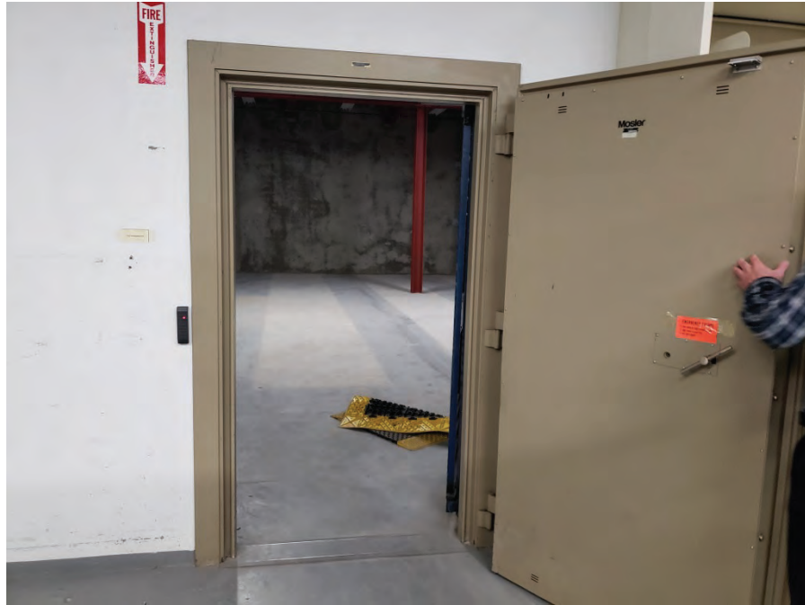
Photograph 5: View of secure room within the warehouse portion of the site.
