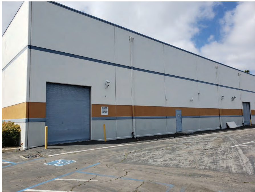
Photograph 4: View of warehouse portion of the site building.
