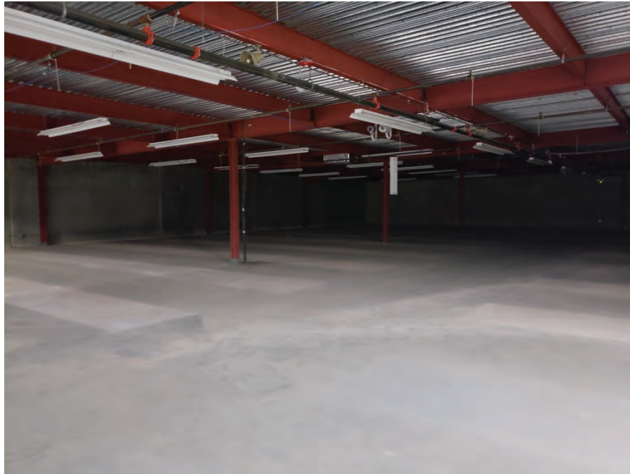
Photograph 7: View of 2 nd floor portion of the warehouse area.
