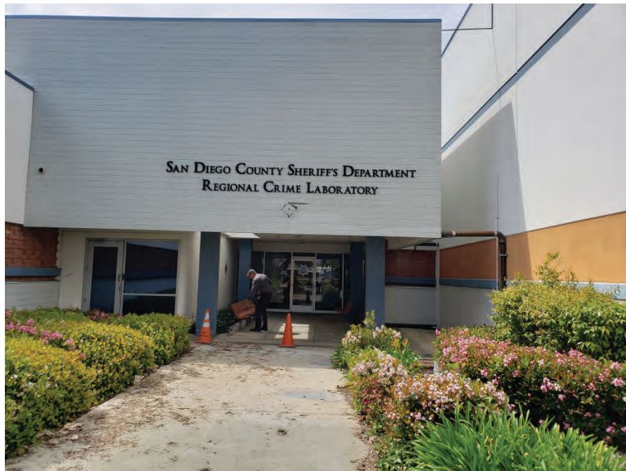
Photograph 2: View of the main entrance to the site building.
