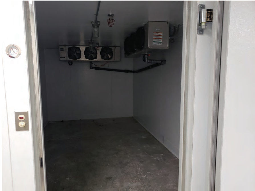
Photograph 27: View of cold storage room within laboratory.
