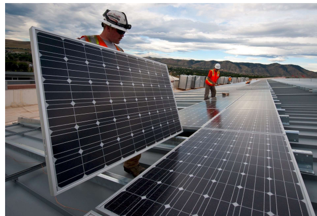
Worker installing rooftop solar panels
