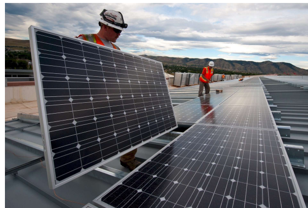
Worker installing rooftop solar panels
