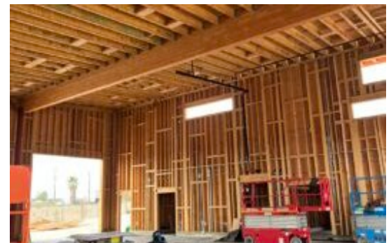
East Otay Mesa Fire Station during construction
